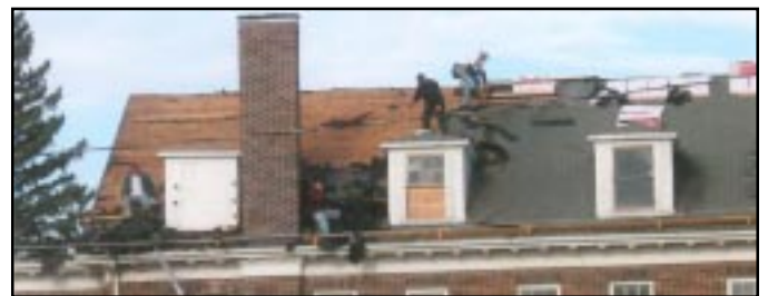
Shingling the roof
