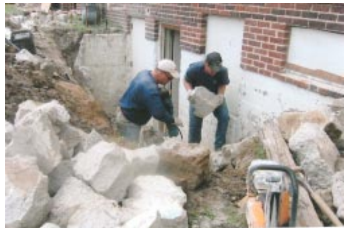
Digging out the old stairs leading to the kitchen
